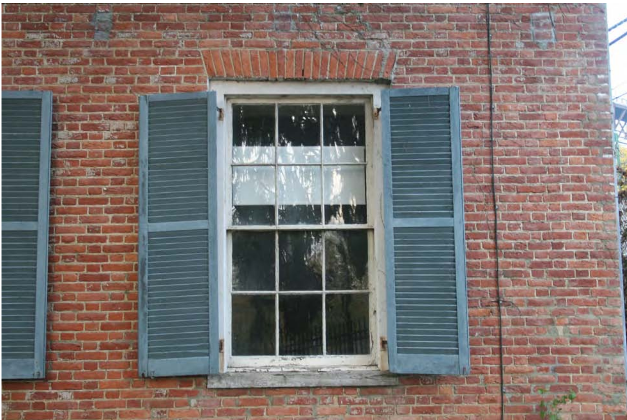
Fig. 20 - Hoffman house, south elevation. Representative example of wood sash and frames, shutters, and brick opening.
