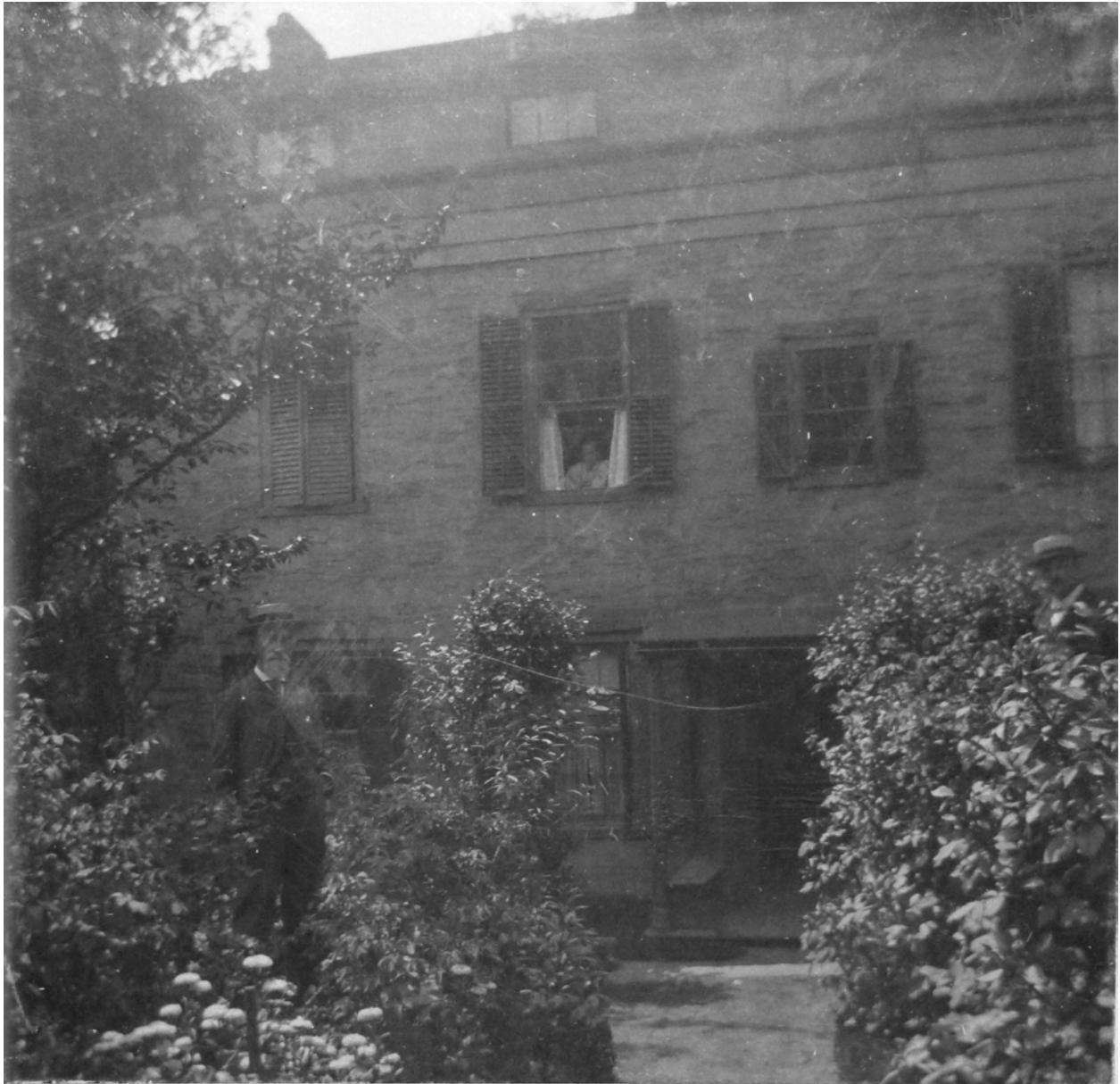
Fig. 44 - Hoffman house. Detail of photograph showing north elevation. Not dated. Smaller stair hall window can be seen at the second floor. Note the covered stoop at the door opening. Also notice the location and design of the windows in the half story. Courtesy of Locust Grove Historic Estate archives.
