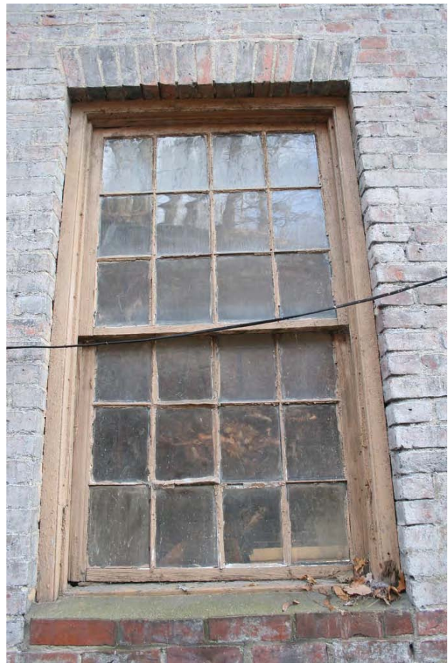
Fig. 64 – Reynolds house. West elevation, second floor. One of two remaining twelve-over-twelve light windows.
