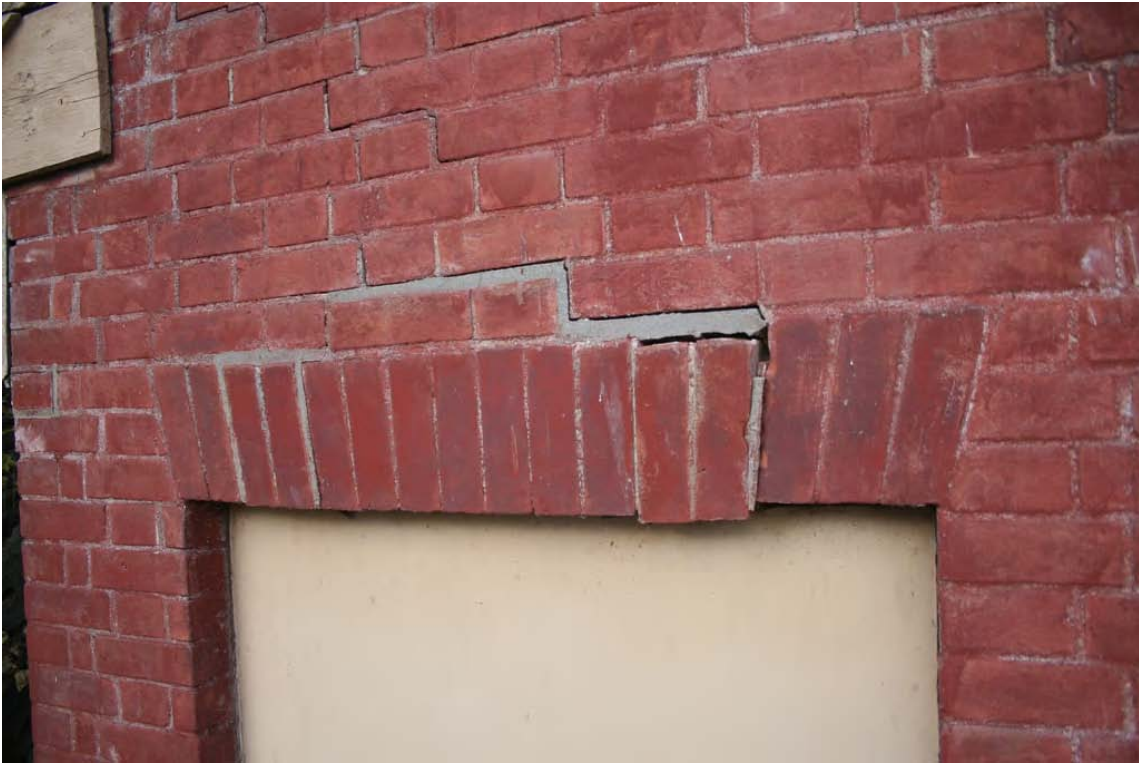
Fig. 62 - Reynolds house. South wing, south elevation. Failed lintel. Past efforts to point the joints display the tell-tale signs of Portland cement mortar. Open gaps indicate the lintel has moved since these repairs were carried out.
