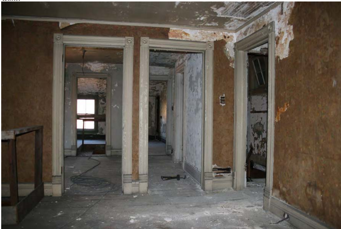
Fig. 38 - Hoffman house. Half-story, southwest room. View looking north. All of the woodwork -- door architraves, corner blocks, base boards -- at this level is late-nineteenth, machine run millwork.
