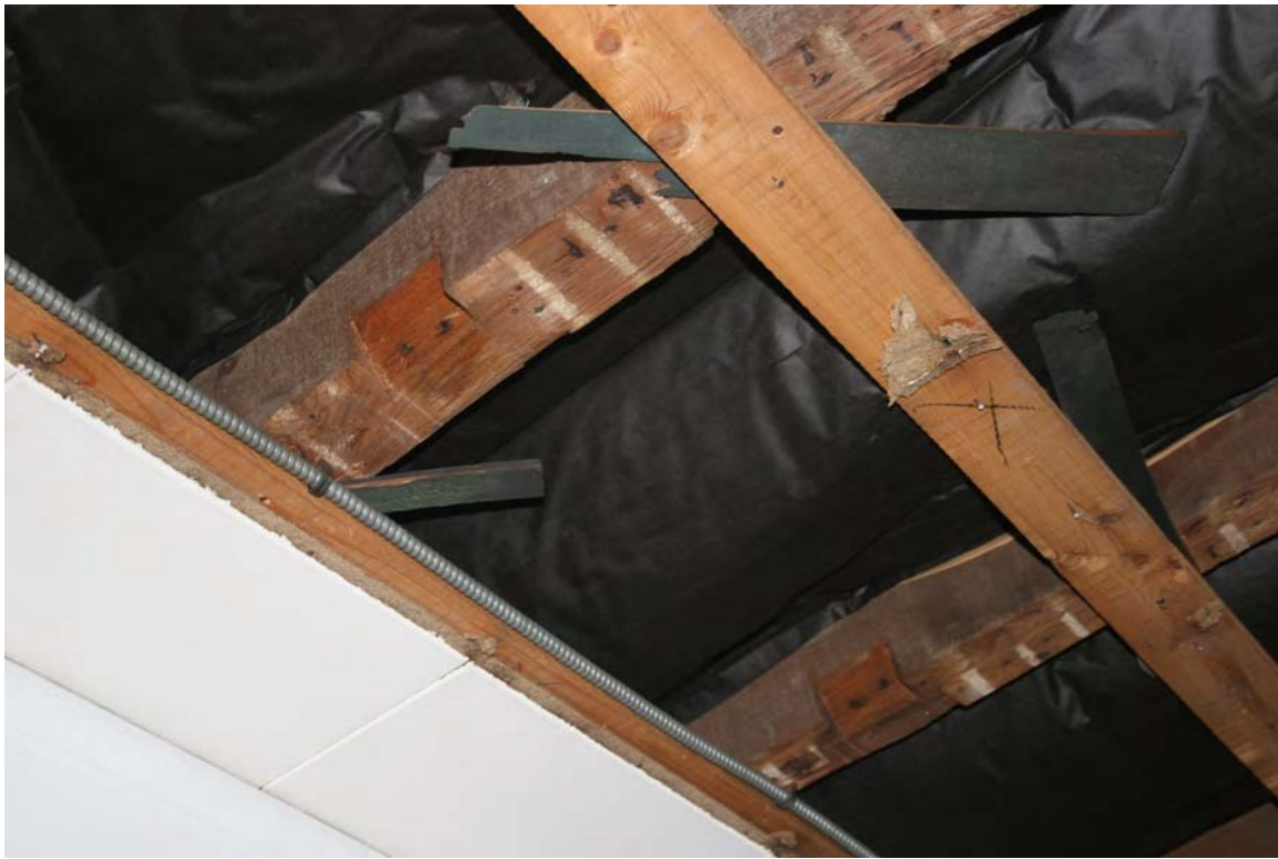
Fig. 37 - Hoffman house. Second floor, west of stair hall, middle room. Bevel cut, lap joints indicate the locations of where earlier stud walls were located. This detail was used throughout the house to frame the walls.
