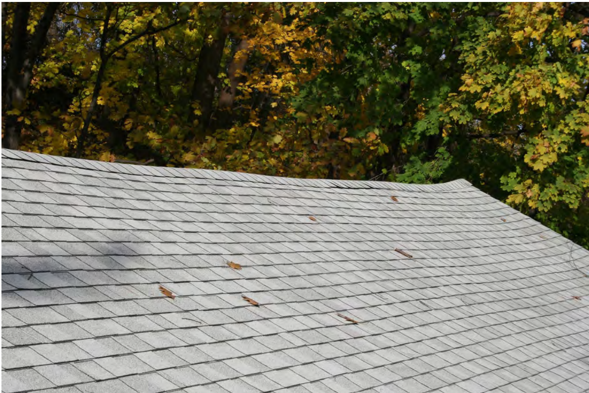
Fig. 57 – Reynolds house. Roof, view looking north. The roofing is in good condition. Note how the roof dips near the far gable.
