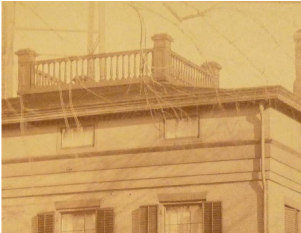
Fig. 41 - Hoffman house. Detail of late-nineteenth century photograph showing roof balustrade. Note the turned balusters. Also notice the design and configuration of the cornice. The leader pipe at the right of the image exists from under the cornice, suggesting a built-in gutter. Courtesy of Locust Grove Historic Estate archives.
