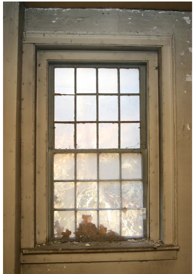
Fig. 47 - Reynolds house. Second floor, west elevation. Representative example of an original, Federal style, single fascia window architrave.
