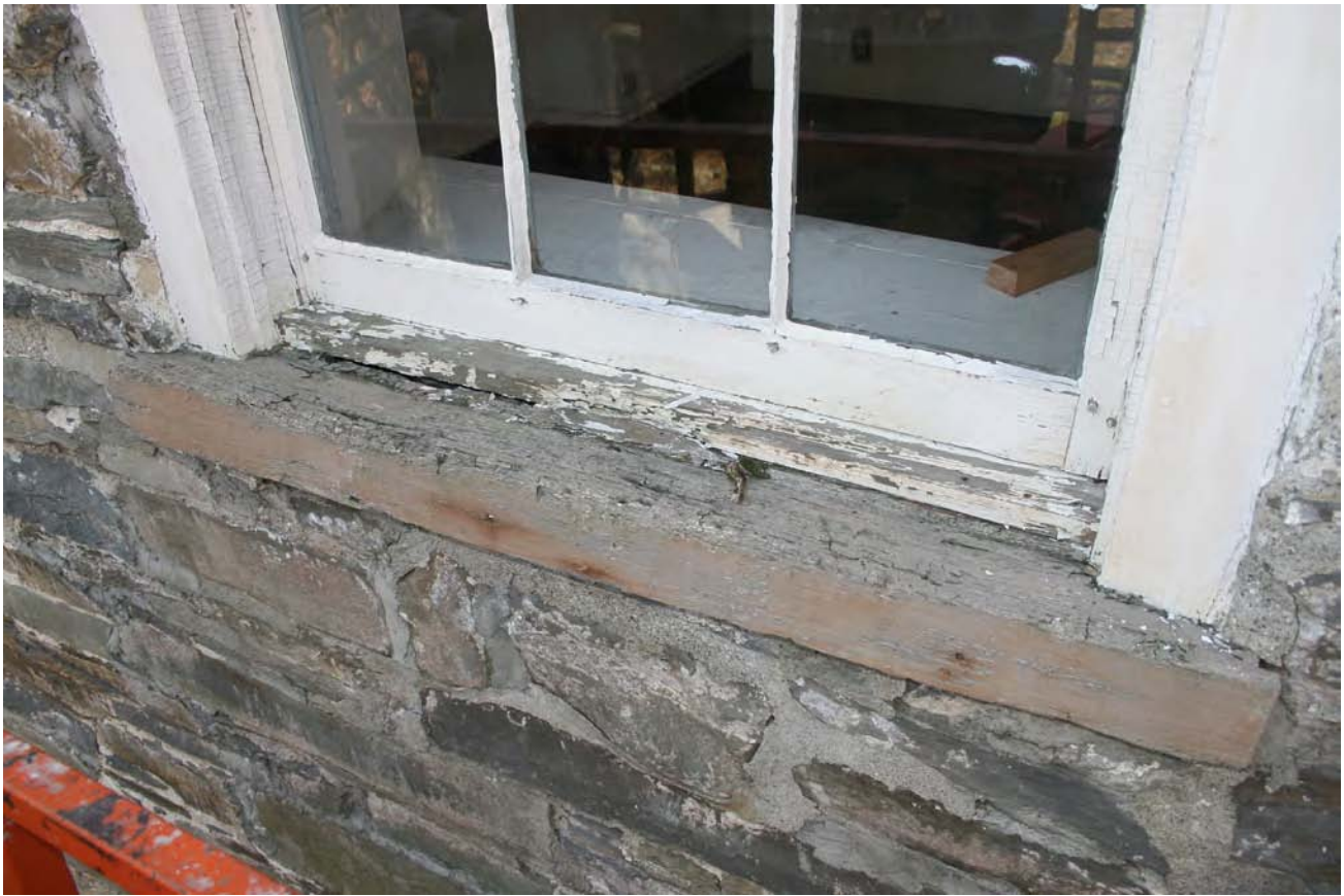
Fig. 42 - Hoffman house. North elevation, second floor. Representative condition of the wood window sills.
