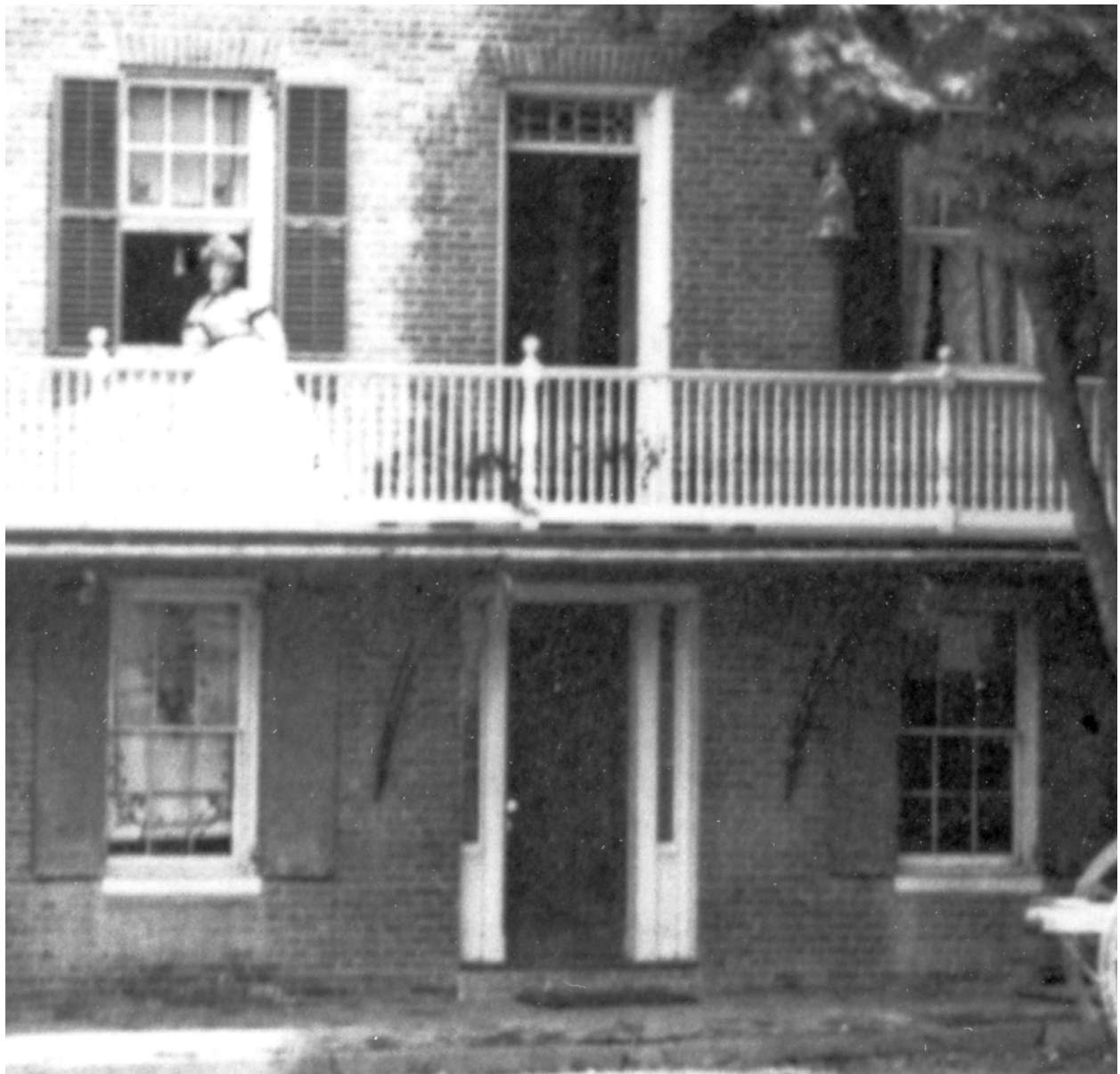
Fig. 67 - Reynolds house. Detail of door and window openings. Note the different door frames and treatments. Notice the decorative transom above the second floor door and the differences in first and second floor shutters. Iron brackets support the second floor porch. The balustrade along the porch has turned posts with turned balusters between.
