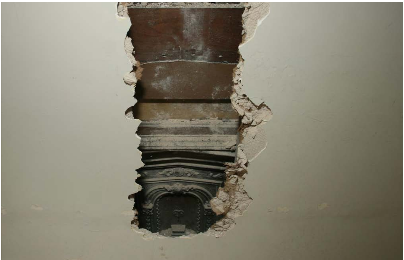
Fig. 30 – Hoffman house. First floor, southwest room. The fireplace opening here contains remnants of a mantel and cast iron insert.
