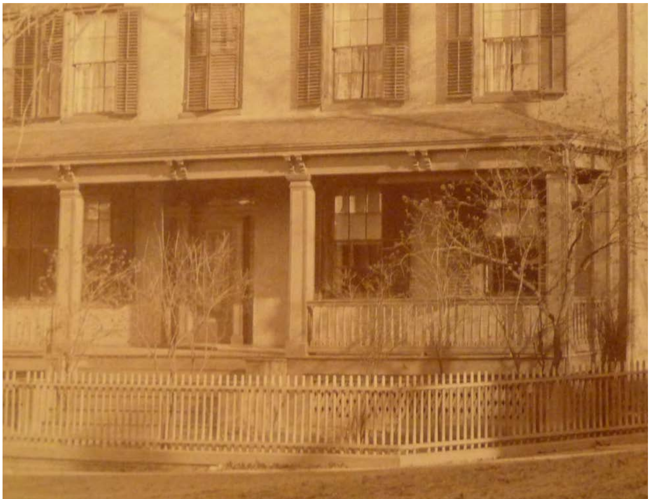
Fig. 46 - Hoffman house. Detail of photograph showing south elevation. Note the porch elements: paired brackets, paneled posts, turned balusters, lattice, and steps. Courtesy of Locust Grove Historic Estate archives.
