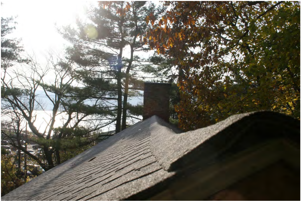
Fig. 58 - Reynolds house. View looking south. Note the saddle in the ridge of the roof.
