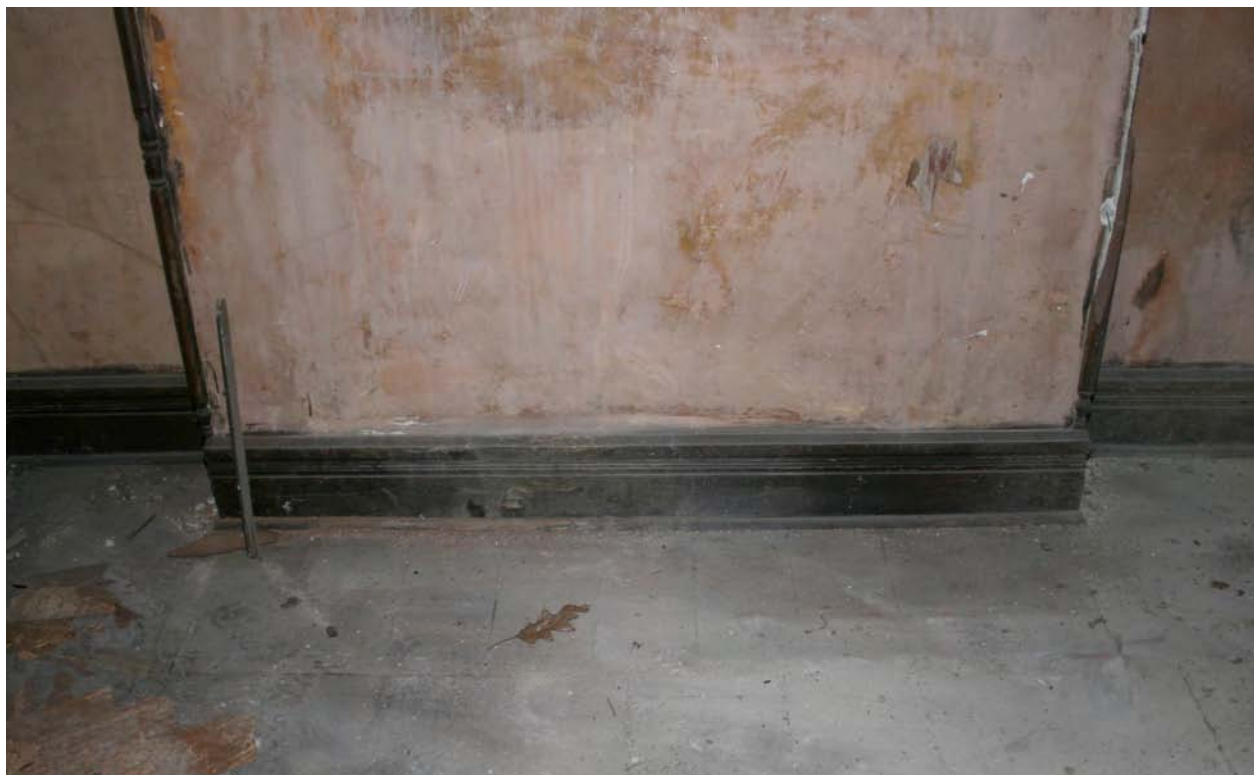
Fig. 55 – Reynolds house. Third floor, north elevation. Detail of patch in flooring where the forehearth of the fireplace extended to. Based on the later finishes, it appears this was removed when the building was renovated into a tenement house.
