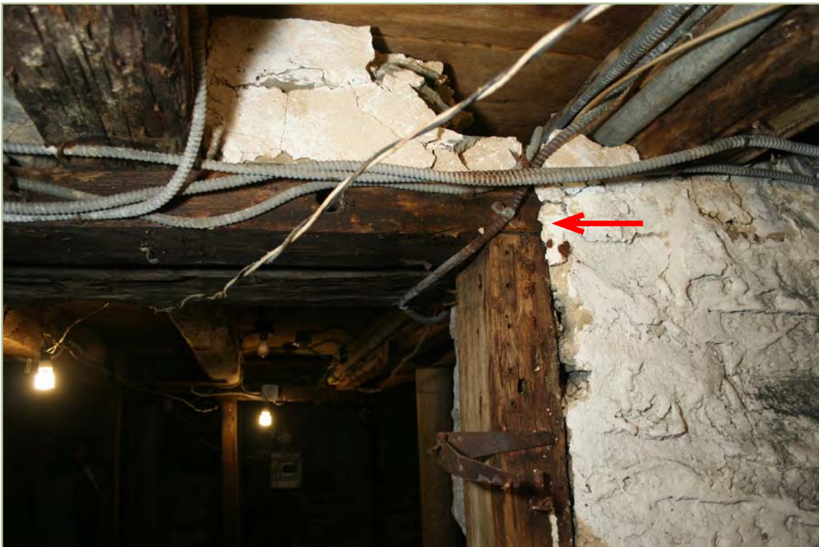
Fig. 25 - Hoffman house, cellar. View looking south. Detail of door frame illustrated in preceding image. Arrow identifies location of joinery used to construct this element.
