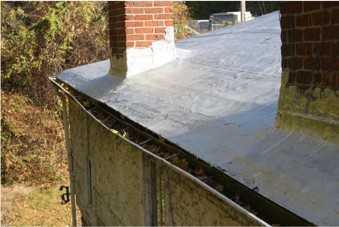
Fig. 40 - Hoffman house. West side of roof. Representative example of coated, built-up roof, chimney flashings, and gutter system. Note damaged gutter filled with leaves, and remains of vines on wood siding.
