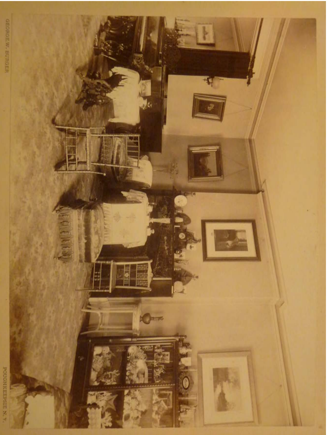
Fig. 29 - Hoffman house. View of the front (south) parlor in foreground and back parlor beyond. The architectural finishes (the mantel, cornice, baseboard) reflect details associated with the Greek Revival style (Gothic Revival in the case of the mantel). Dated January 19th, 1897. Courtesy of Locust Grove Historic Estate archives.
