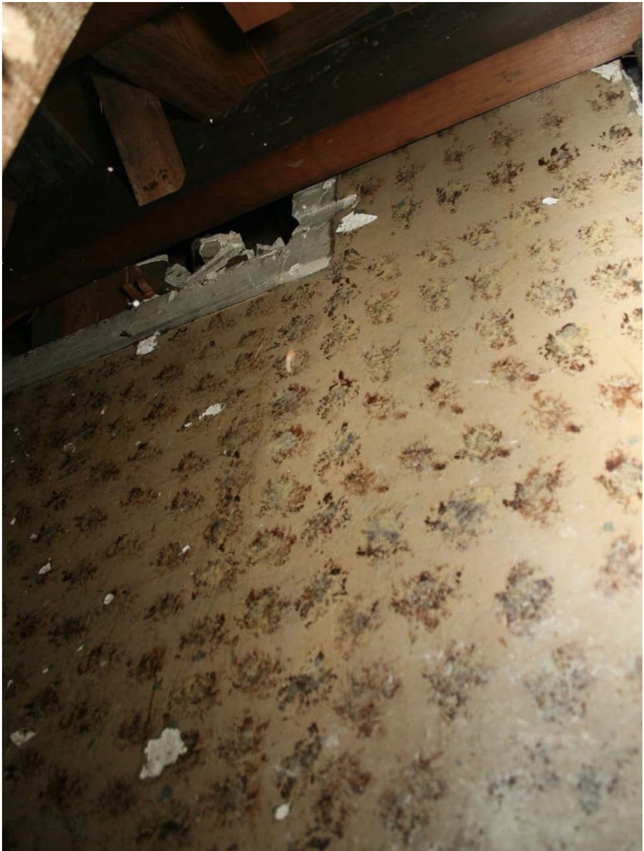
Fig. 31 - Hoffman house. First floor middle room. A large portion of the earlier plaster wall remains buried behind the existing west wall of the room. The unpainted plaster at the top of the image is where a window architrave and apron was located. The wall is painted with an early rag or sponge applied finish.
