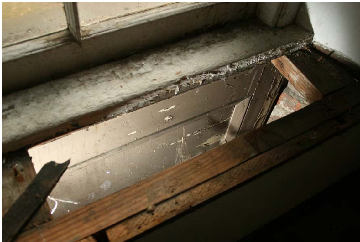
Fig. 32 - Hoffman house, second floor, southeast room. Recessed panel with flattened quirked ovolo located under east window opening.
