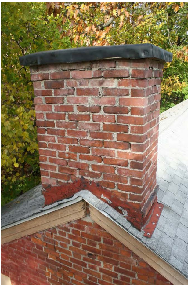
Fig. 60 - Reynolds house. South chimney of main roof. This chimney as well as the end wall below need rebuilding. Note deteriorated condition of brick and mortar, flashing and wood trim.
