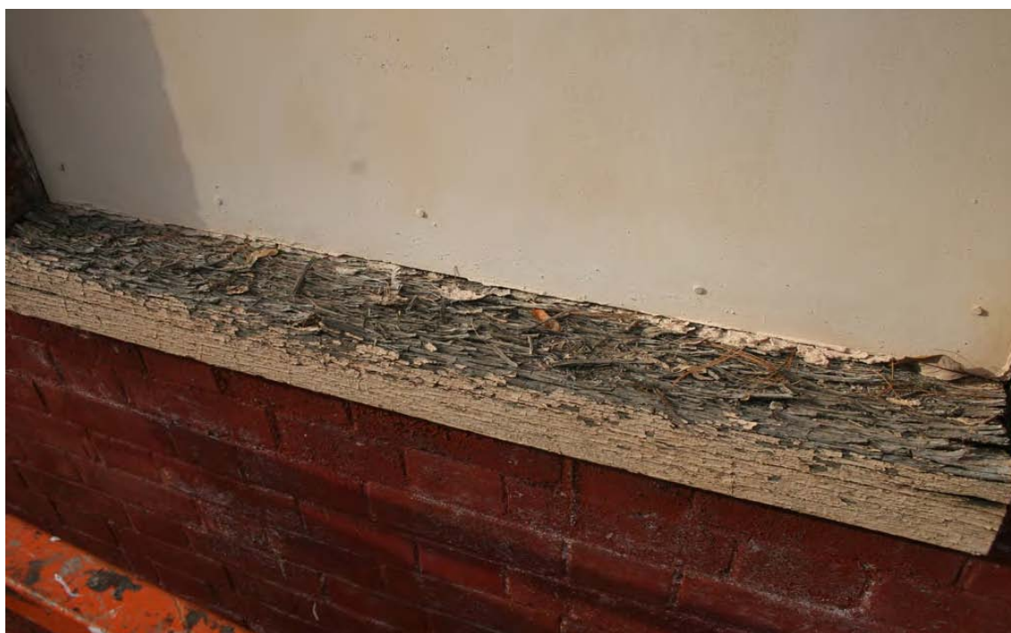
Fig. 66 - Reynolds house. Representative example of the deteriorated condition of the wood window sills.
