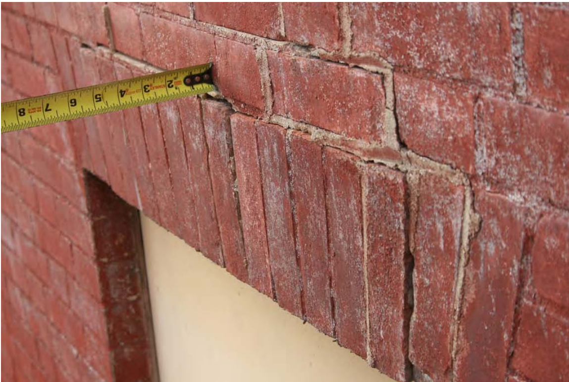
Fig. 63 - Reynolds house. East elevation, second floor. Detail of failing lintel. Bricks has dropped and shifted resulting in open joints.
