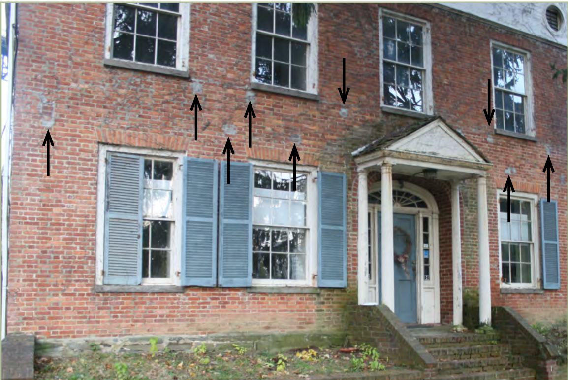
Fig. 22 - Hoffman house, south elevation. Areas of patched brickwork where framing for the porch roof was located.
