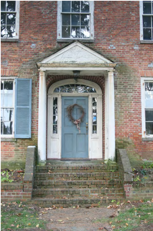
Fig. 18 – Detail of the Colonial Revival entry and portico. The masonry opening was altered in the early twentieth to accommodate the Federal style door surround. The portico is believed to be contemporary with the door opening or added shortly after.
