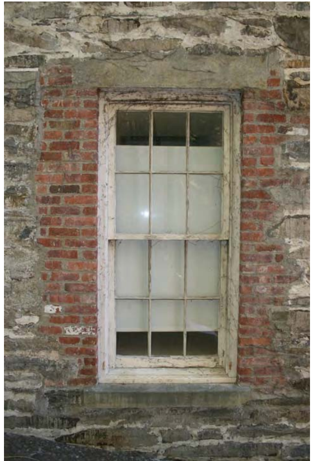
Fig. 19 – Hoffman house, west elevation. Typical example of a later window opening introduced in the stone masonry. This alteration was performed in the Twentieth century. The sides of the opening are built in brick set in Portland cement mortar and the lintels and sills are formed in concrete. Note the dimensions of the sash compared to those found on the south elevation (preceding image).
