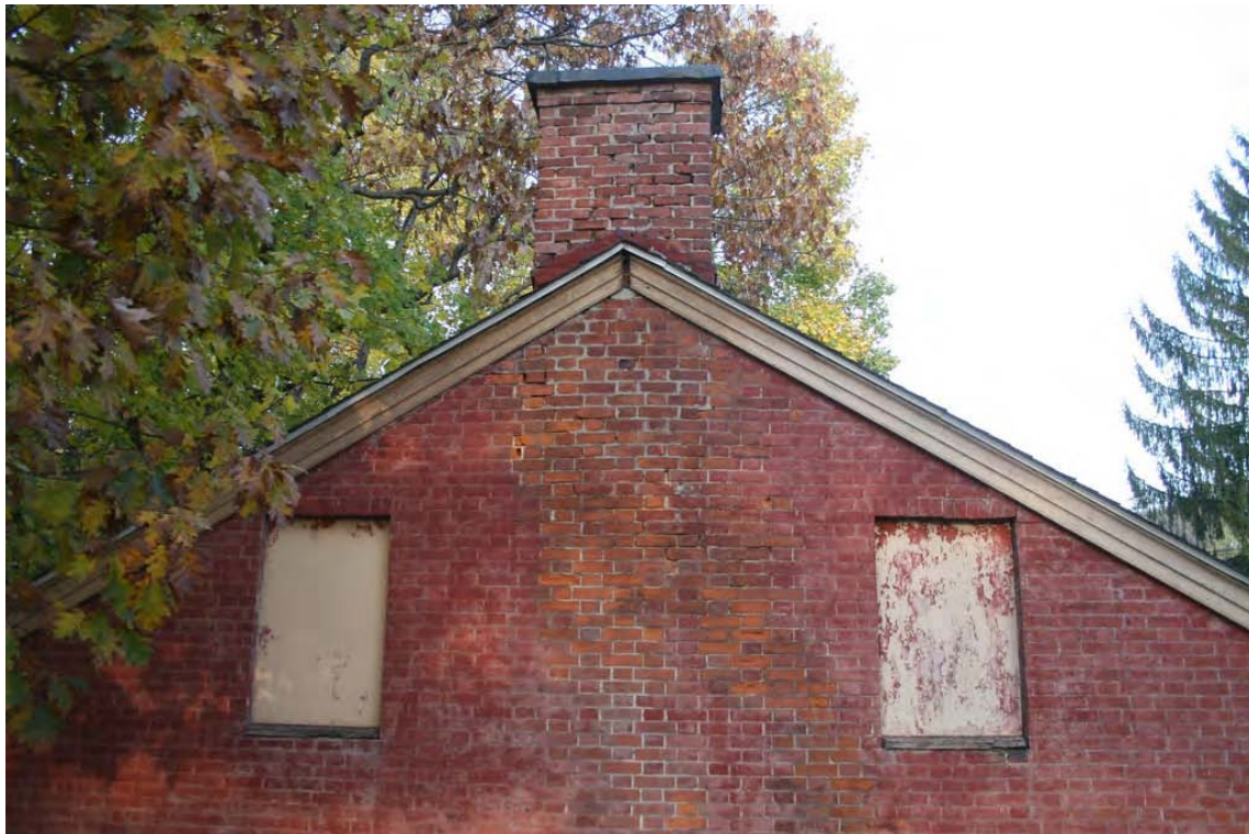
Fig. 59 - Reynolds house. South elevation. The brick along the path of the chimney flue is deteriorated and needs pointing and selective rebuilding.
